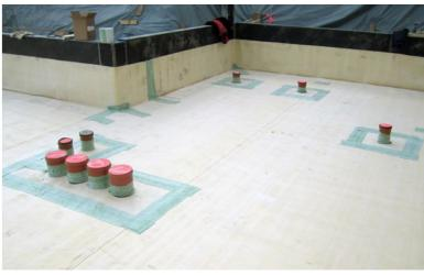
Finished internal jointing detail
