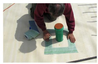
Internal jointing detail with SikaProof® Tape-150
