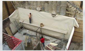
Walls, single or double faced formwork
