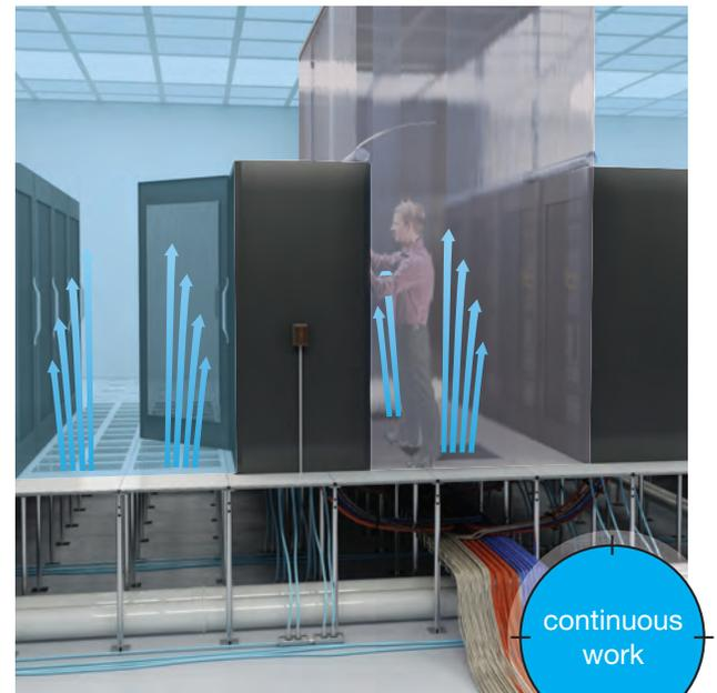
SmartAire T provides on-demand cooling lowering temperatures in a contained hot aisle allowing the technician to safely work on equipment in the aisle for an extended period of time.
