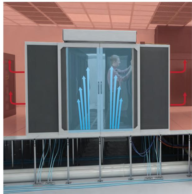
SmartAir P monitors the static pressure differential from the contained cold aisle to the hot aisle in order to maintain a balance when rack loads vary. This balance reduces bypass airflow through servers, racks and other containment structures.
