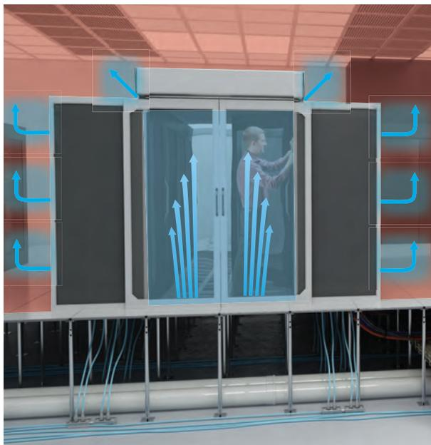
Without SmartAir P Dampers in the cold aisle to maintain a neutral static pressure in the cold aisle, conditioned air will leak through idle servers and other gaps in the containment structure.
